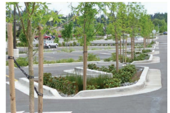
Figure 4-17. Rain gardens, a Low Impact Development solution to parking lot storm water management in Charlotte, NC
